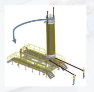
Once ready, the finished stack is then tilted using powerful cranes
